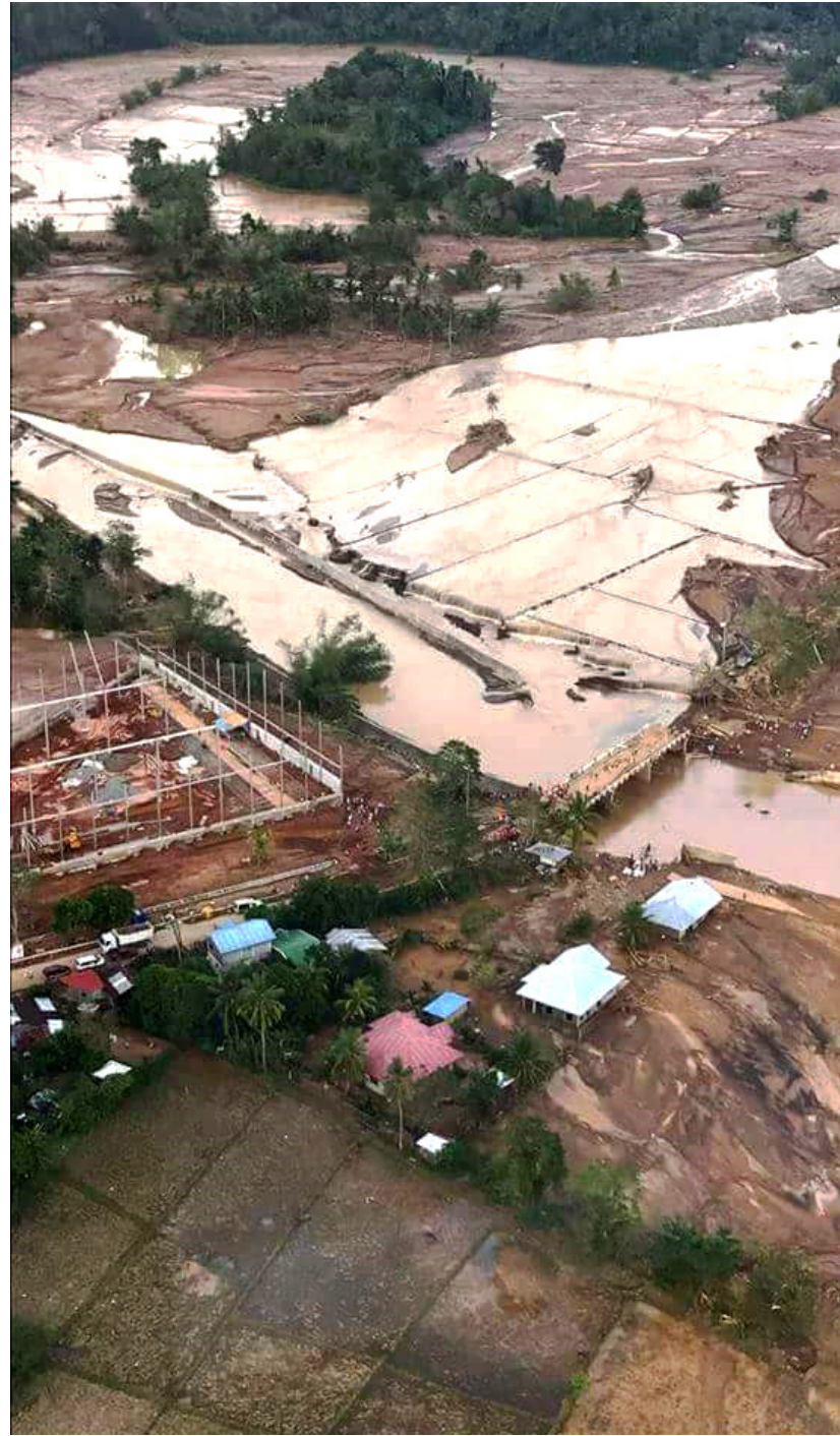
The massive volume of floodwaters from the mountains destroyed the grandeur of nature and all the infrastructures and facilities along its path carving new geographic landscapes as it receded.
