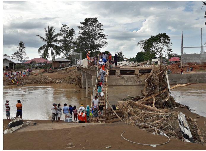
Pedestrians had to wait in queue before braving to cross this makeshift ladder made of wooden electric pole.
